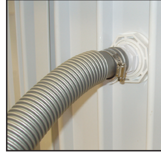
Figure 17 — Free end of hose attached to return
