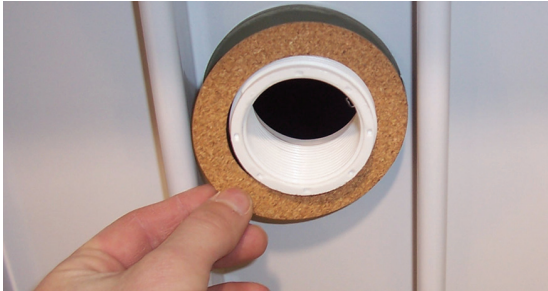
Figure 5 - How to install rubber & cork gasket outside
