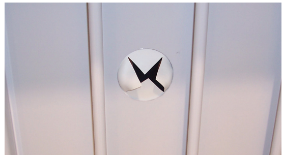
Figure 2 - Liner opening cut
