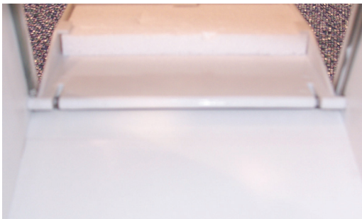
Figure 14 A - View from inside of skimmer
