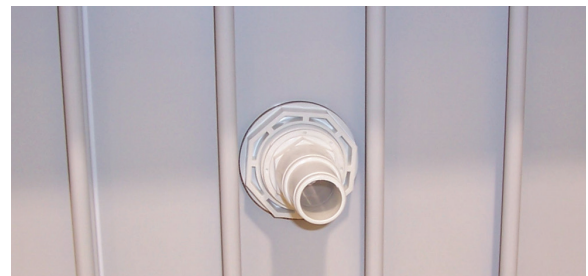
Figure 11 - Return with outside return fitting
