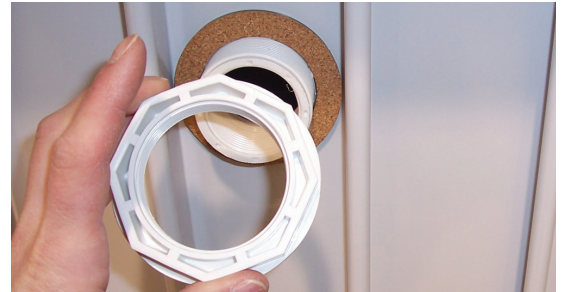
Figure 6 - Locknut
