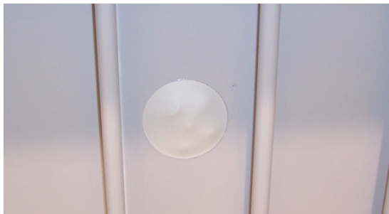
Figure 1 - Liner against wall
