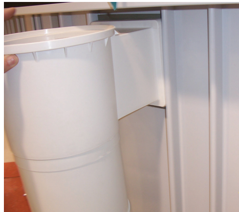
Figure 4 - Lining up skimmer body with gasket
