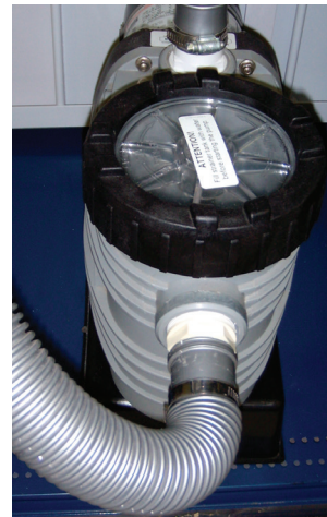
Figure 12 - Attaching hose to pump
