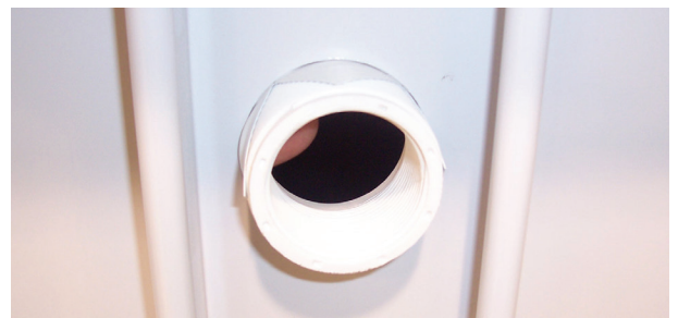
Figure 4 -Return pushed through wall
