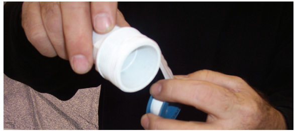
Figure 7 - Applying Teflon tape to hose adaptor
