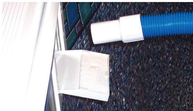
Figure 3 - Positioning weir for vacuuming
