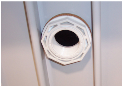
Figure 7 - Direction locknut should face
