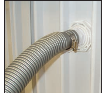
Figure 17 — Free end of hose attached to return
