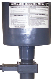
Figure 15 – Slide valve installed in bottom of skimmer
