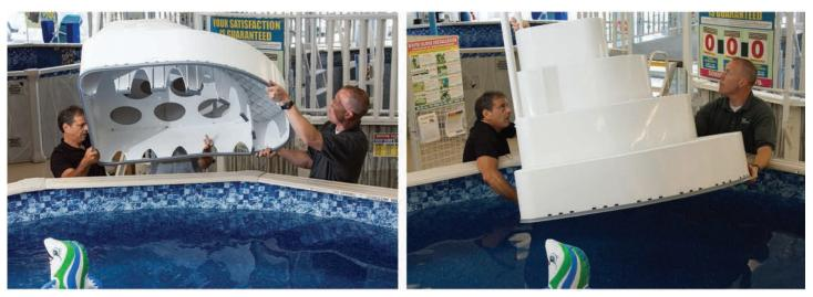
Carefully lift the step over the pool top rail and gently lower the step into the pool. This will take a few minutes since the trapped air in the step will need to escape through the vent holes as the step lowers into its final position.
